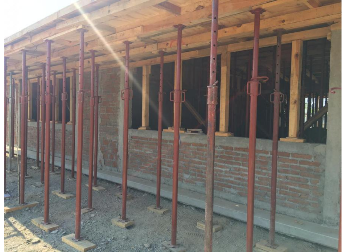
Timber concrete falsework with metal propping
