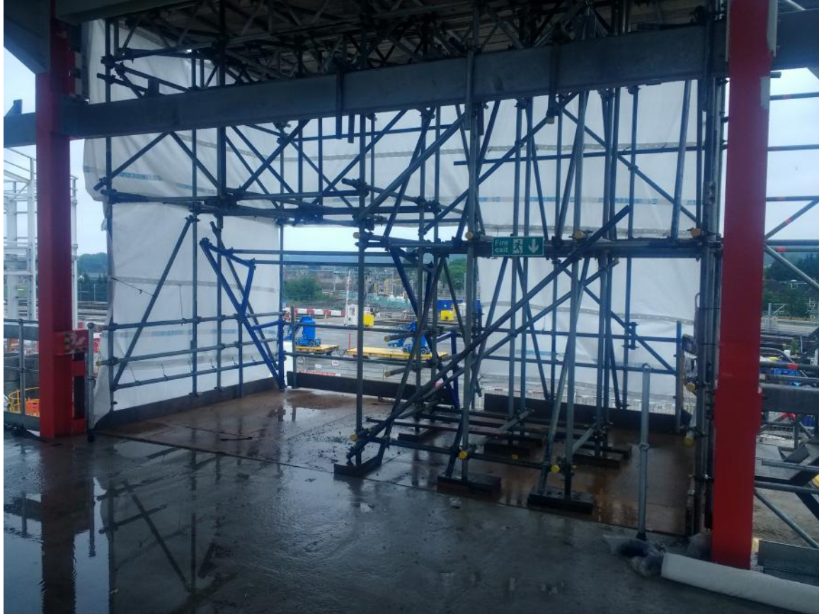
Scaffold loading bay and access
