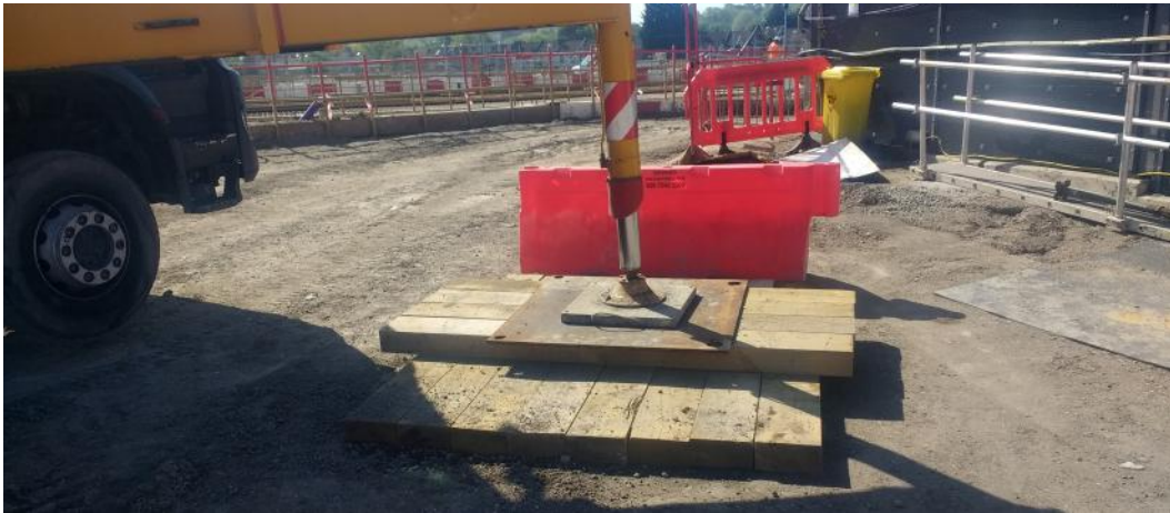
Temporary plant loading on permanent works
